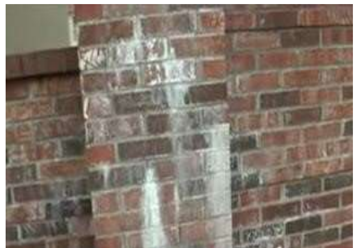
EFFLORANCE ON BRICKS
